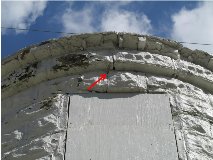
Photo 5: Step Crack at West Elevation
